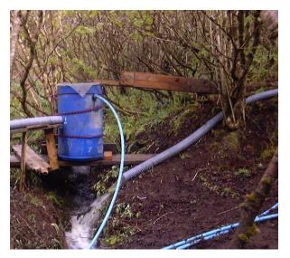
This blue plastic barrel is not a thing of beauty but it functions well as an intake. A means of scouring the silt out of the barrel would be a useful addition. There is room for improvement in the way the overflow is handled, though. It would be best to collect the overflowing water and pipe is safely back into the stream along with any fish that may be carried along.
