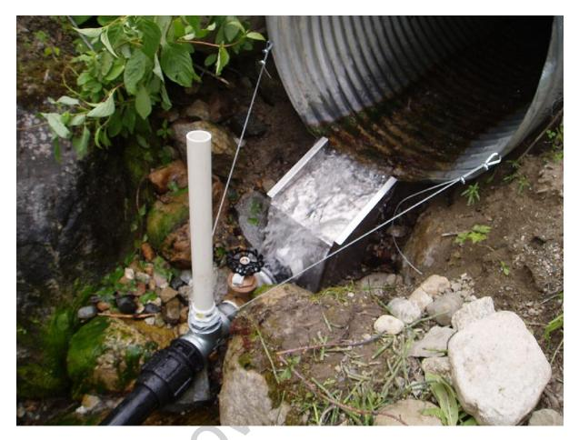
In this example above you can easily see the shut-off valve and the vent pipe. However they are somewhat inaccessible in the event of flooding, and it is actually likely that the vent pipe would be damaged by debris flying out of the culvert.
