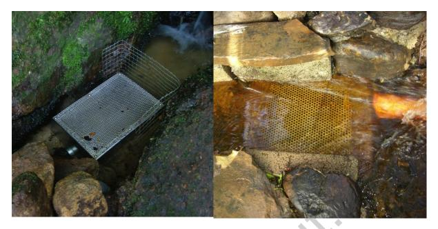
Sometimes the tank can be buried in the stream bed, so that there is no need for any sort of dam or weir structure. All you need are a few stones on each side to direct the flow over the screen.
