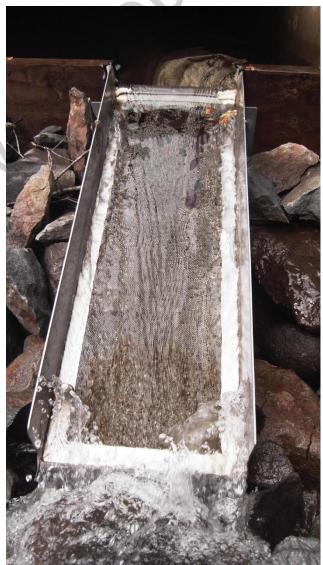
These photos below show screen boxes built into various sorts of dams. Water flows over the lowest part of the lip of the dam/weir and down the filter screen. In the event of a flood there is a wider spillway available for the flow.
