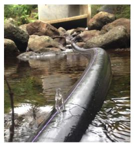
If water stops coming out then any vent at this location will draw air in, which is not normally helpful. In this situation you may have to locate the vent pipe further down the slope where the pressure has built up due to the extra head.
